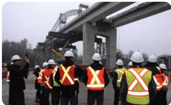
Burgoyne Bridge, St. Catherines
